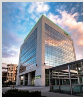
HQ Mansion of DKV, Spain
